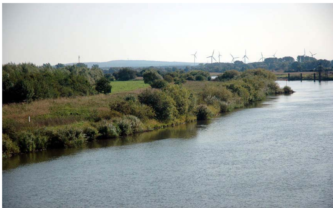
Figure 9: Biotechnical bank stabilization at Stolzenau (from: Bauer, BfG, 2006)
