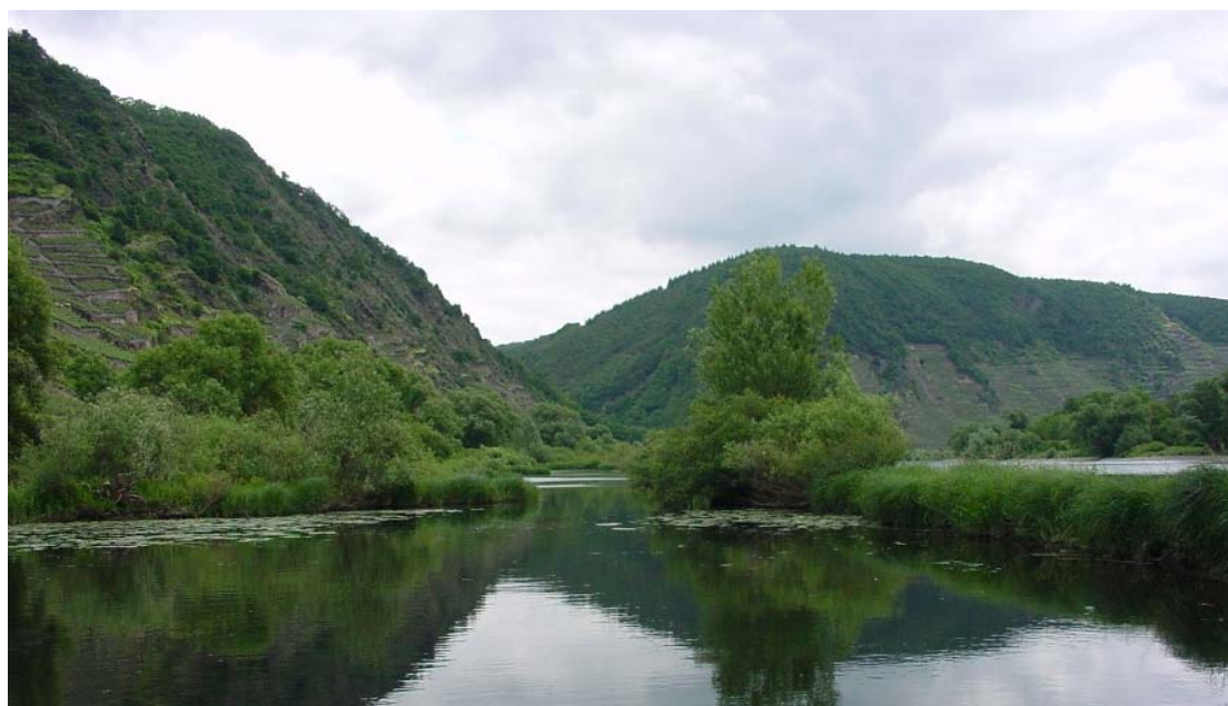
Figure 6: Groyne fields behind a parallel structure at Koborn-Gondorf (from: von Landwüst, BfG, 1999)
