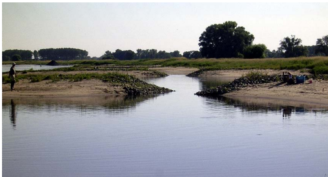
Figure 8: V-notch groynes in the River Elbe (from: Anlauf, BfG)
