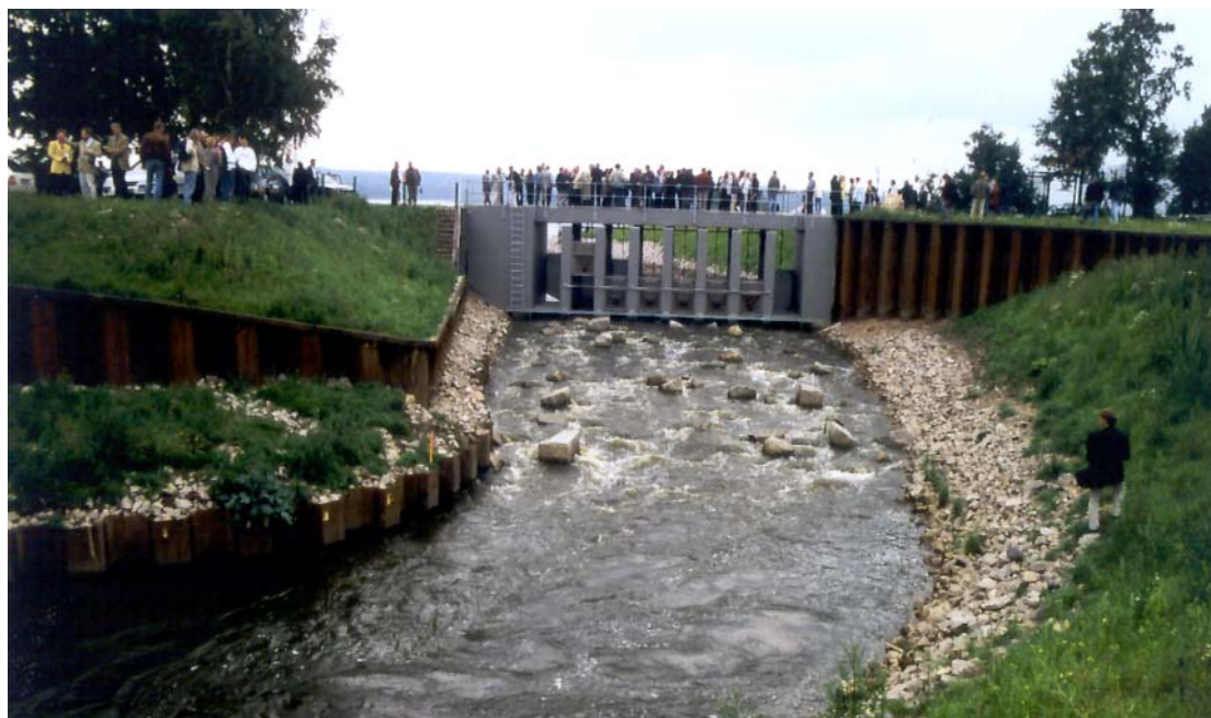
Figure 5: Nature-like by-pass channel at the weir Geesthacht/River Elbe (from: Nöthlich, BfG, 1998)
